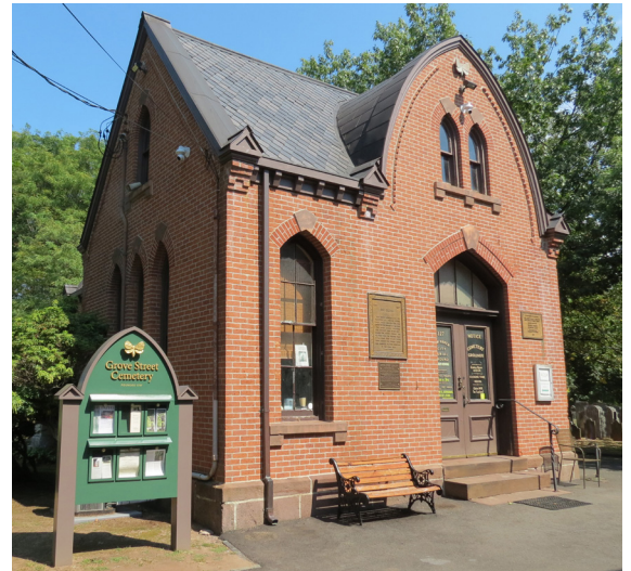
The attic over the office held surprises including records of the building's design by New Haven architect Rufus G. Russell and its construction in 1871. The new information kiosk stands at left (see story on page 3).
